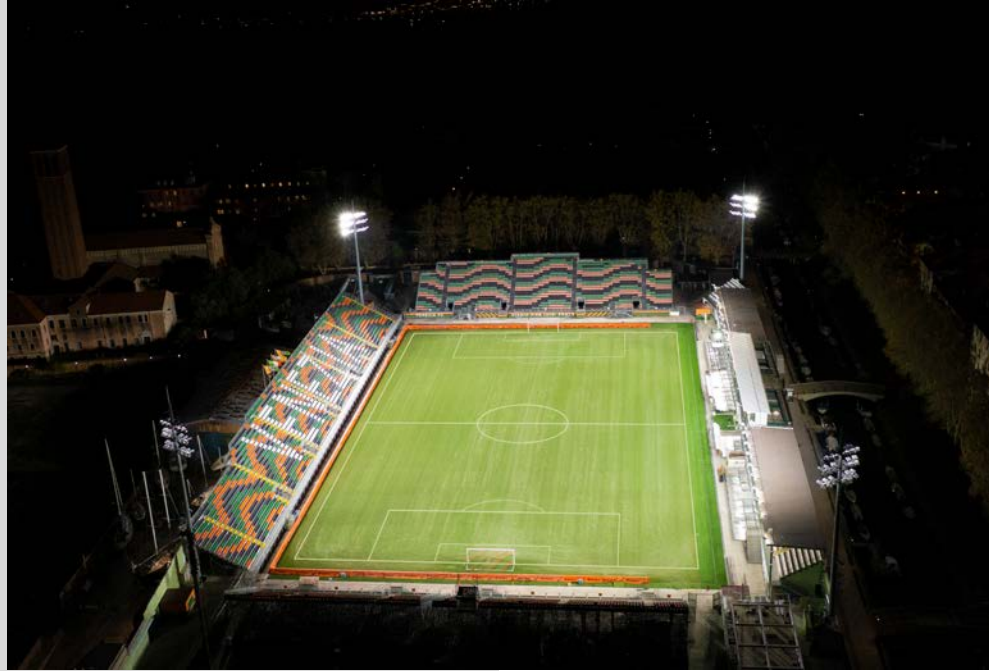
Picture during installation - Pier Luigi Penzo Stadium
