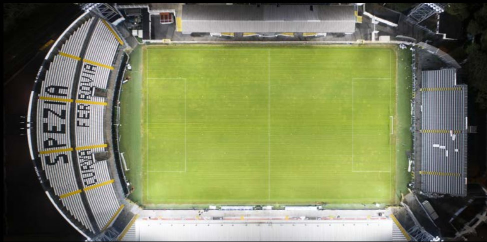
Picture during installation - Alberto Picco Stadium
